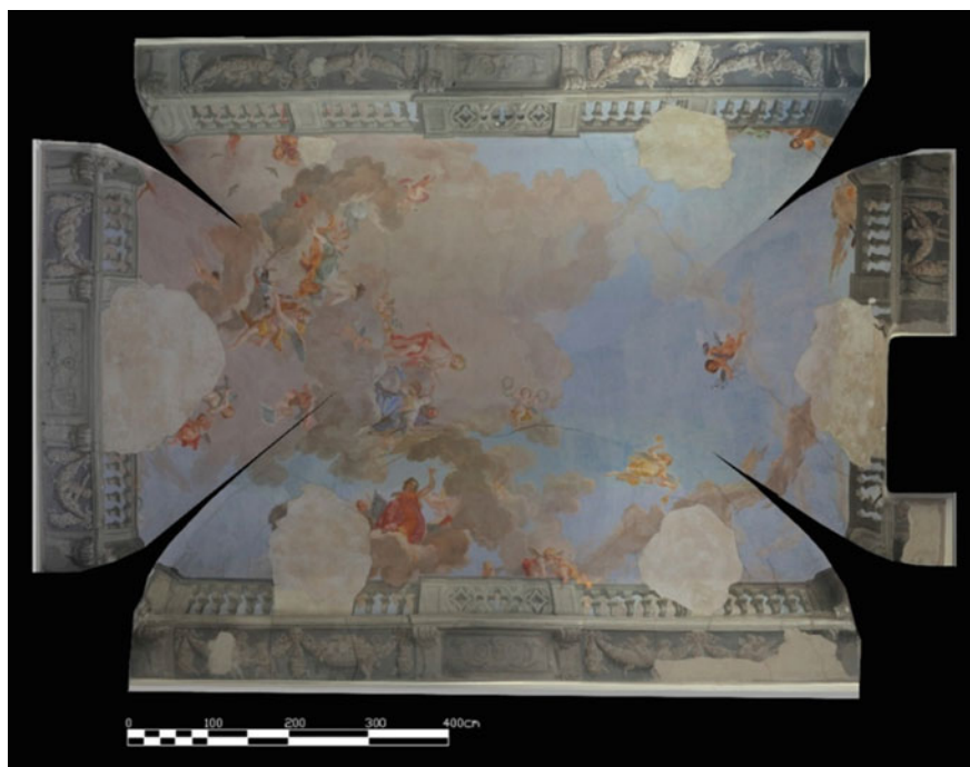
Fig. 13 Planar development of the frescoed vault
